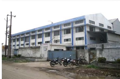
Plant buildings with gates and guard post
