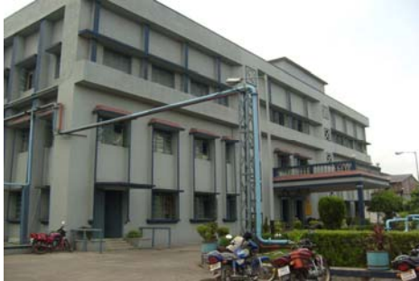
Front entrance to the main building
